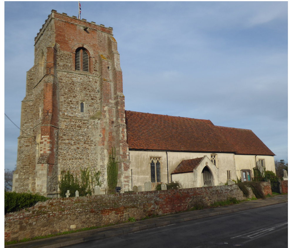
Figure 5 View of Church of St Michael
